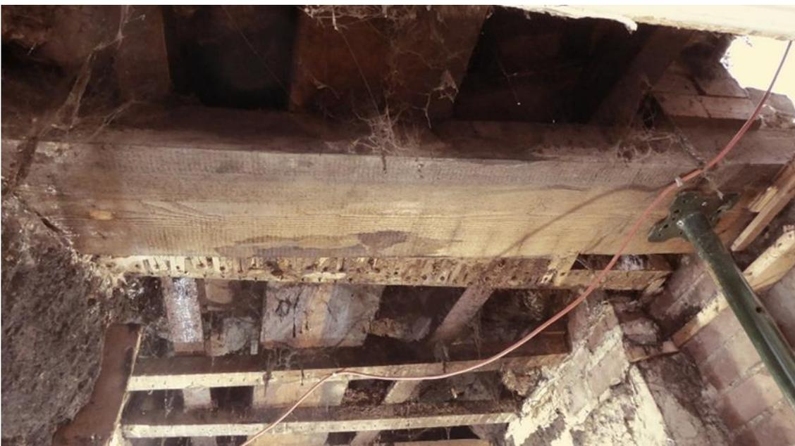
This discovery and subsequent investigations of all the structural issues in several places, the associated calculations and design work will have added around 6 months to the restoration timetable. To make the structurally safe significant reinforcement, blockwork and steel beams will be added.
